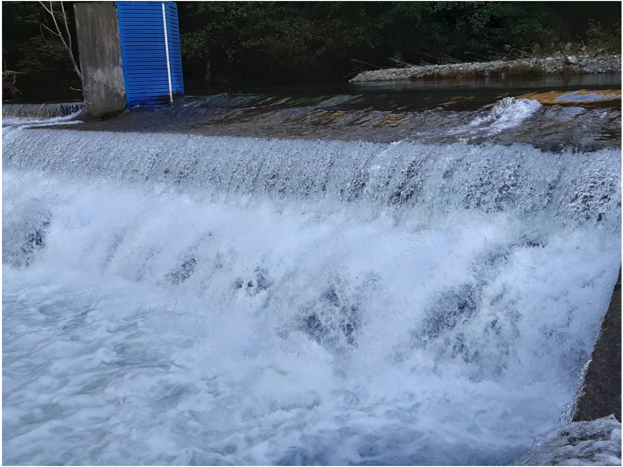
Figure 23. Dam on Chakvistiskali River
