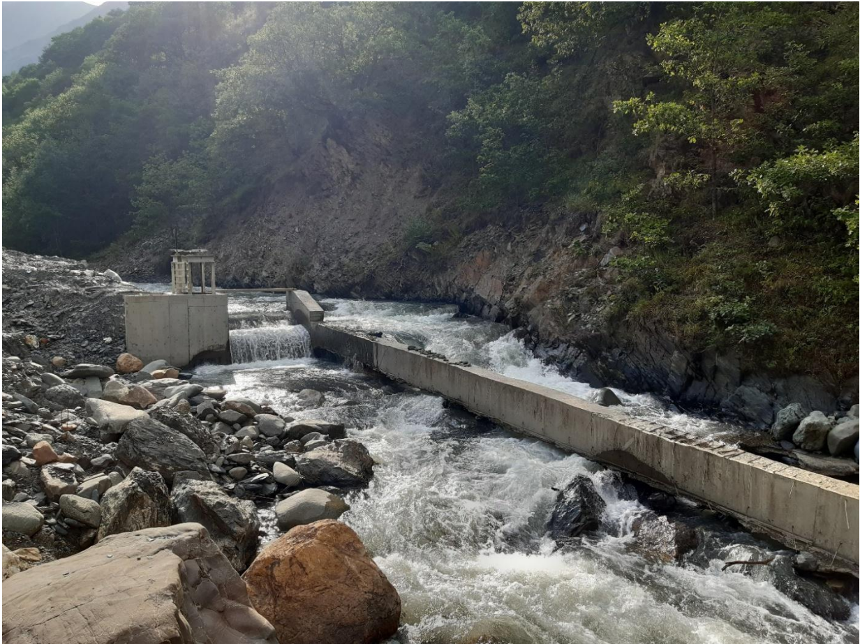
Figure 24. Hydroelectric power stations on Arguni River
